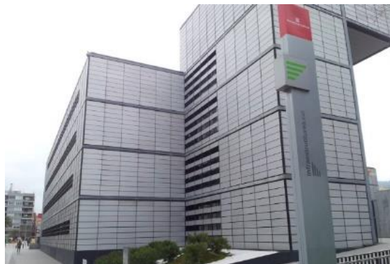
Figure 15. Infraestructures de la Generalitat de Catalunya headquarters building
